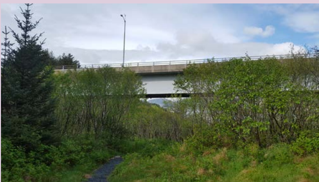
Image 7: Trail (on Near Island) passing beneath the Near Island Bridge
