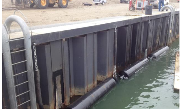
Dock repairs including lighting, ladders, and installation of fender camels.
