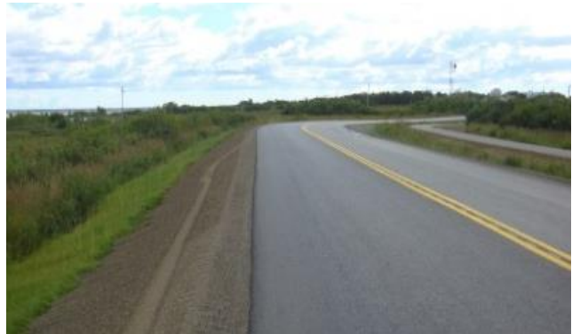
Bristol provided engineering and planning services for the Toward Road Project located in Dillingham Alaska. Collaboration between the Curyung tribe, the City of Dillingham, to ensure all stakeholders were involved in the process.
