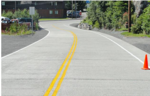
The Shtax'heen Roadways Improvement Project in Wrangell, AK, addressed local concerns about the high number of pedestrians using the route, including children going to and from school.
