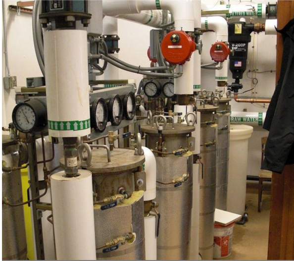
Surface Water Treatment Plant Upgrades in Nondalton, AK.
