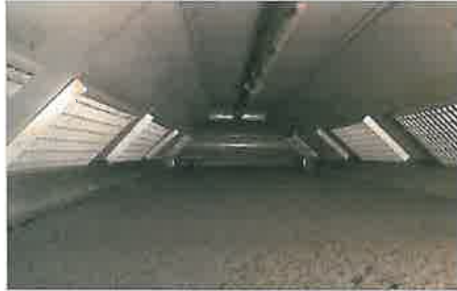
FIGURE 7 Biosolids traveling through the Andritz Belt Dryer
