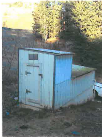
Utility outbuilding for diesel storage
