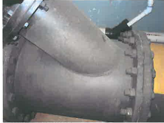
Fabricated steel fitting
