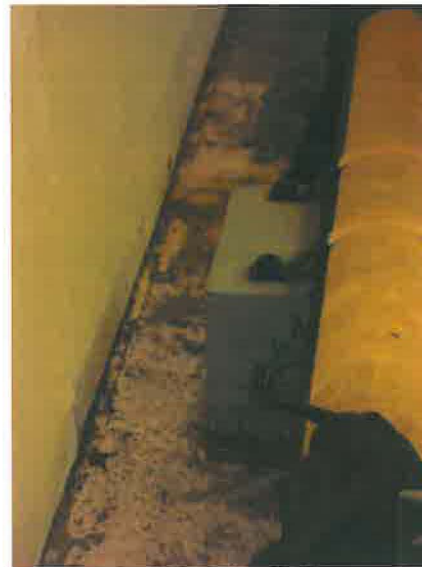
Floor/wall at Machine Hall
