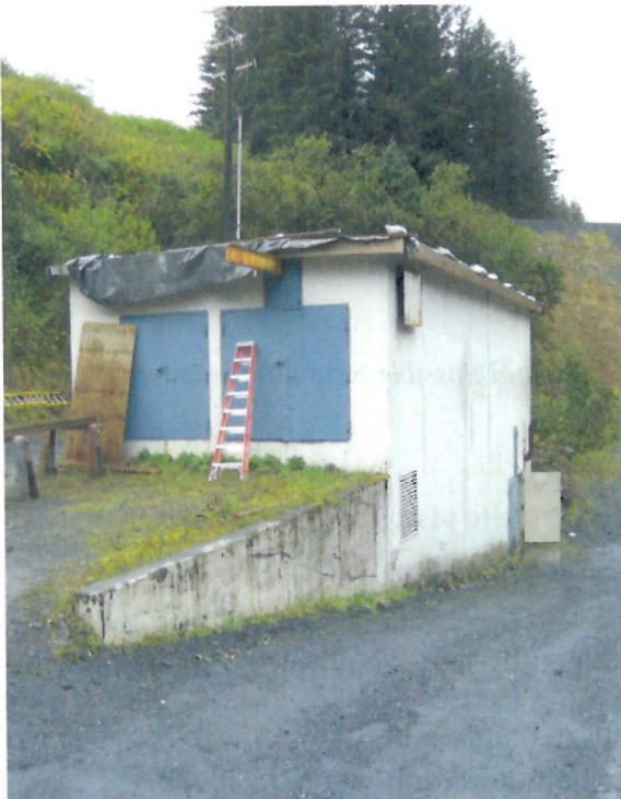
Monashka Pump House – Early 1970's Construction
