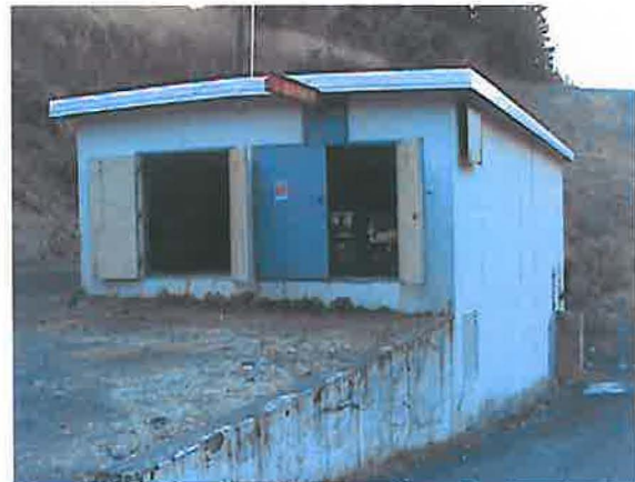
Overall facility view from northeast, showing fluoride and container storage rooms
