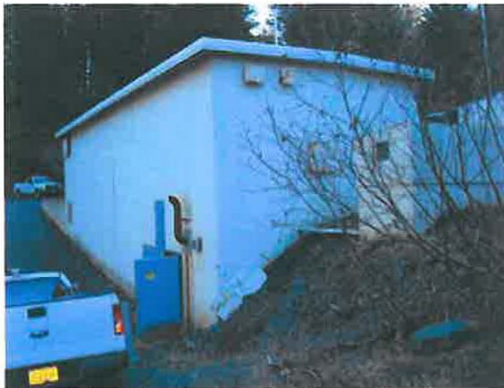
Overall facility view from northwest
