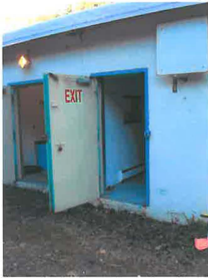
Upper level doors at south wall
