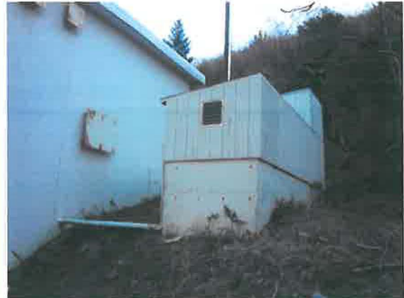
Fuel storage outbuilding
