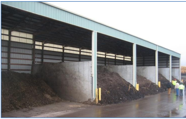
Figure 1 - Aerated Static Pile Bays
