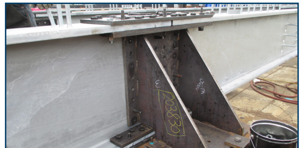
Splicing plates fit up on beams.
