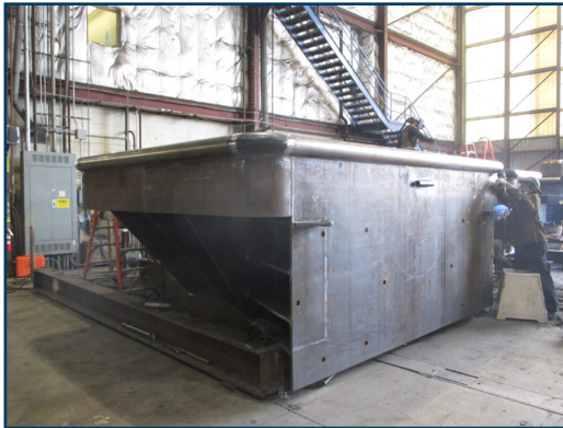
Bullrails welded to perimeter and end plates on cap.
