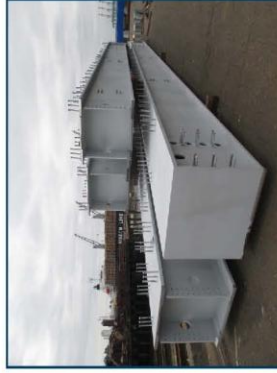
Box beams for grids P25 and P26 waiting for fit-ups in yard.
