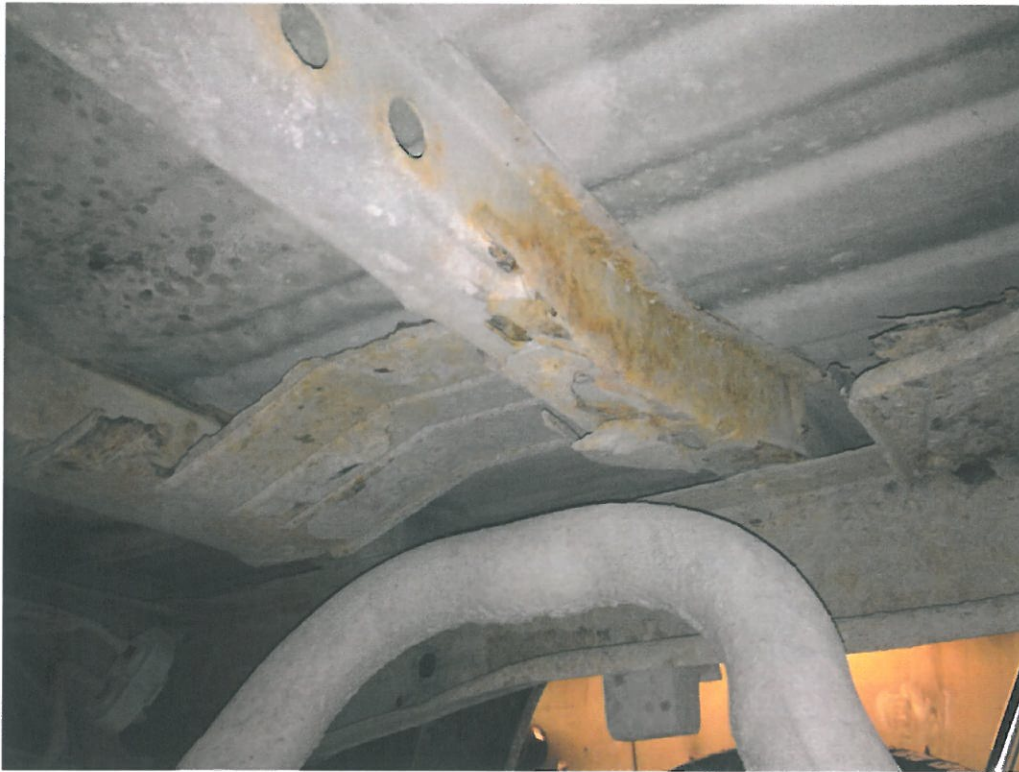
Bed supports rusted through
