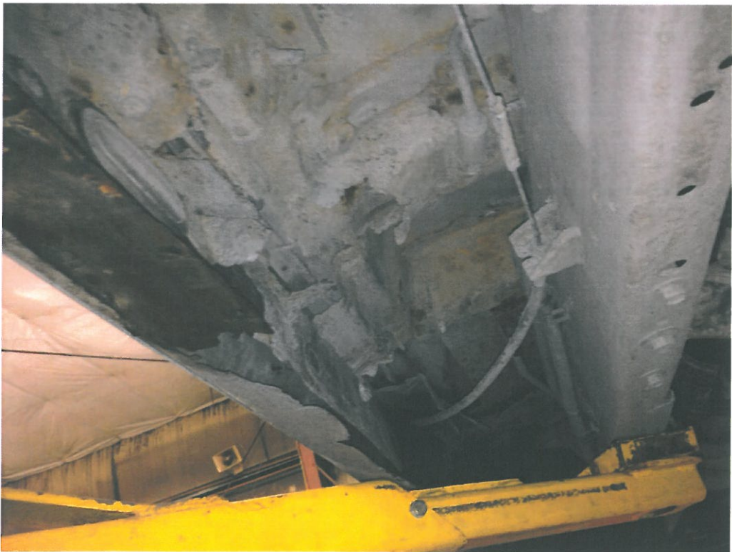
Cab rusted through, drivers side
