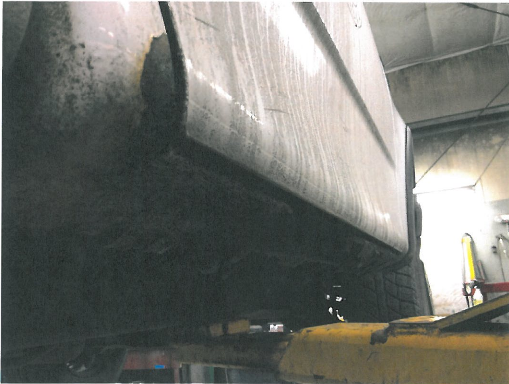
Cab rusted through, passenger side
