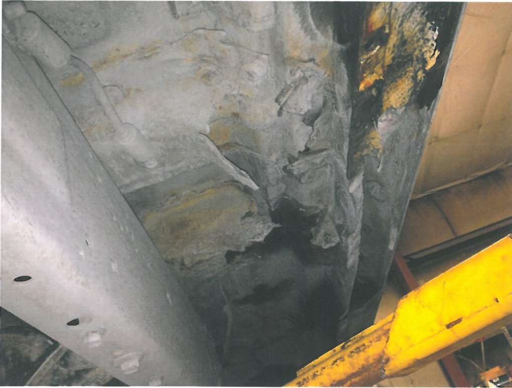
Cab rusted through, passenger side
