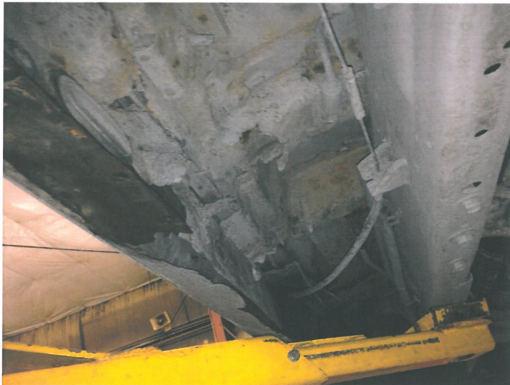
Cab rusted through, drivers side
