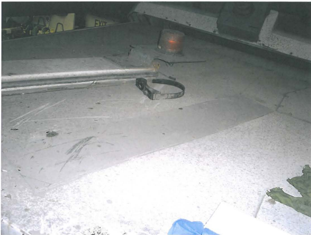
Patching where the hopper roof is worn and rusted through.
