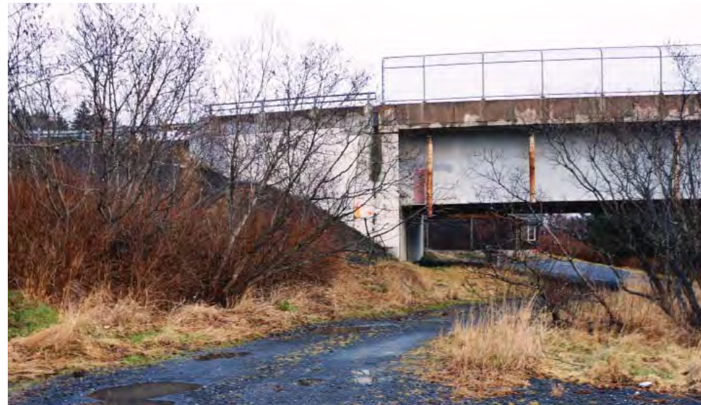
Image 29: Approach to the west side of the bridge.
