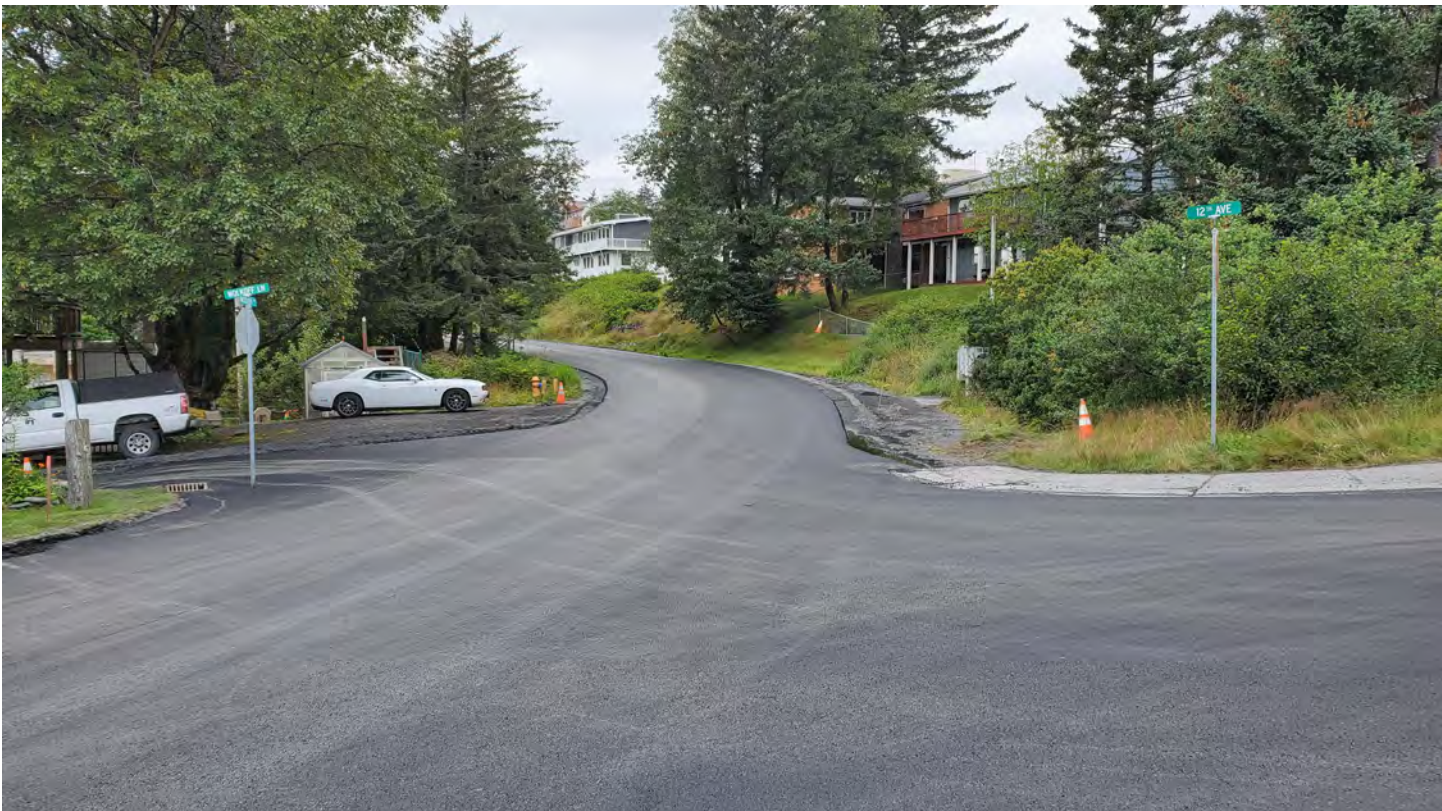
Mission Rd - New pavement
