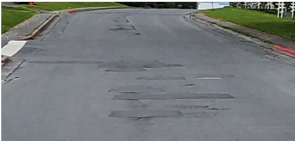
Pothole patching on (Upper) Mill Bay Road, 2021
