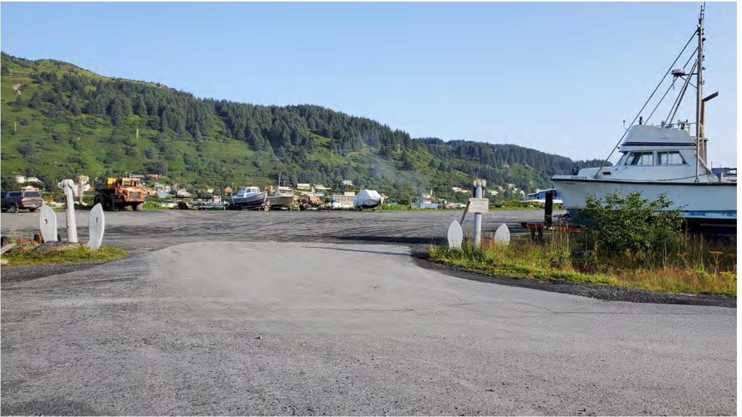
Saint Herman Harbor - Trailer parking (gravel)
