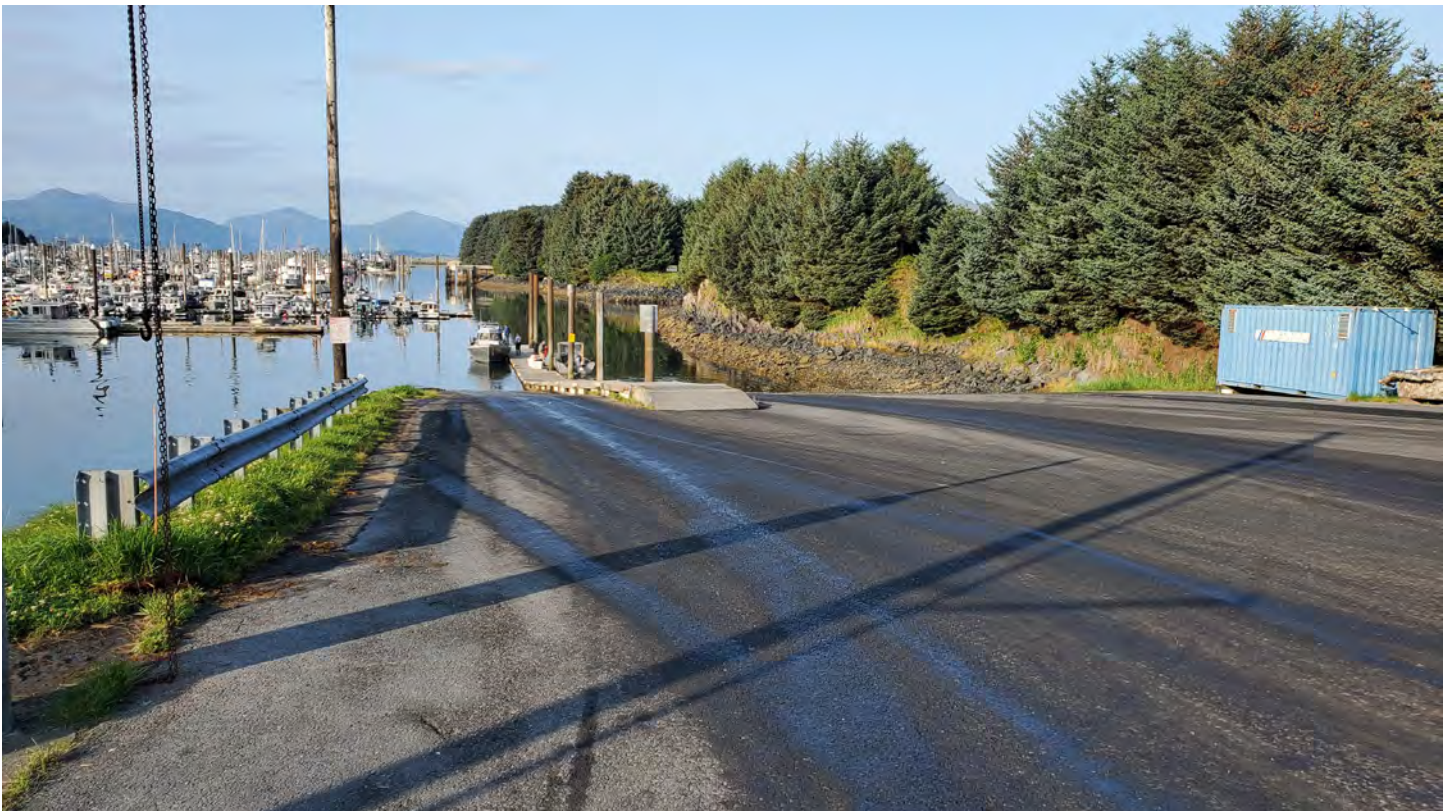
Saint Herman Harbor - Boat launch ramp
