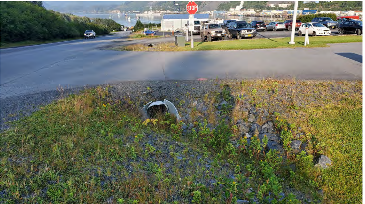
Amilaq Drive - Road culvert
