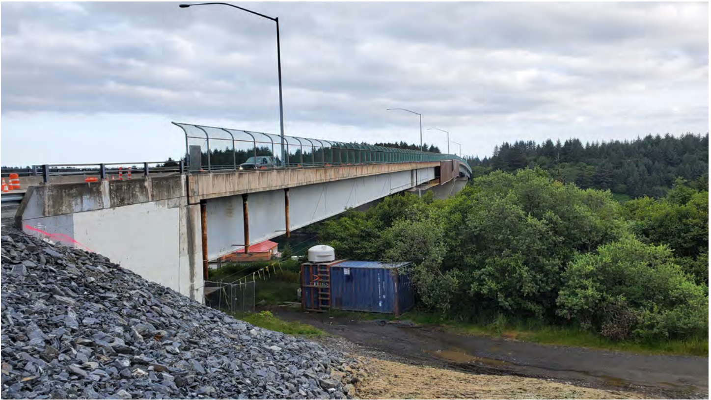
Fred Zharoff Memorial Bridge
