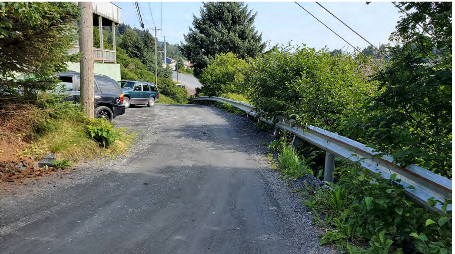
East Hillcrest St
