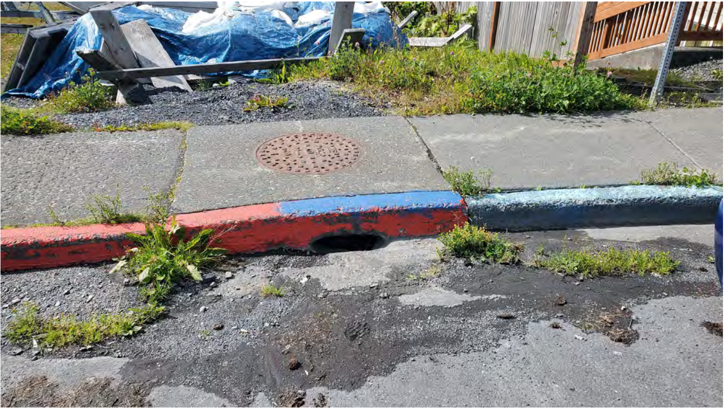
Kashevaroff Ave Storm Drain
