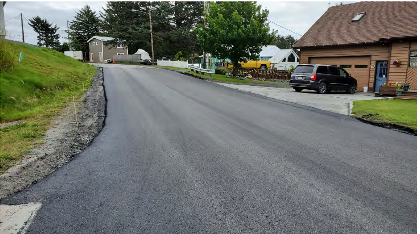
Mission Rd - New pavement (looking east)
