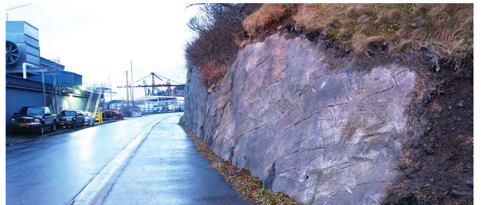
Image 2: Sidewalk constructed along Shelikof Street from Pier 2 to Jack Hinkle Way.
