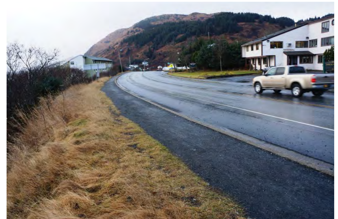
Image 31: Existing gravel edge along Rezanof Drive. View from the bridge looking west on Rezanof Drive.
