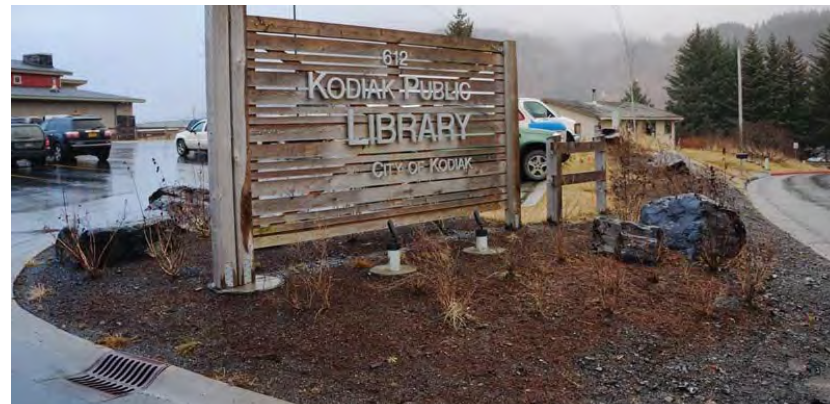
Image 20: Library entry sign. Proposed Sidewalk would wrap right in front of sign.
