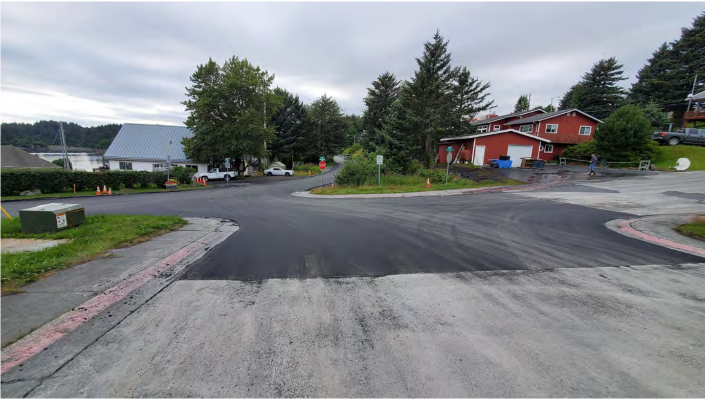
Mission Rd - New pavement (from Ismailov)
