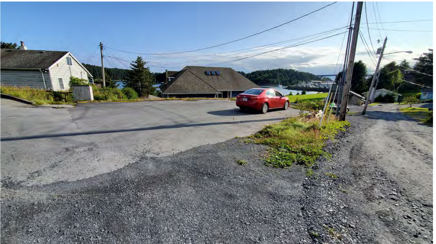
Wolkoff Lane - Paved parking area
