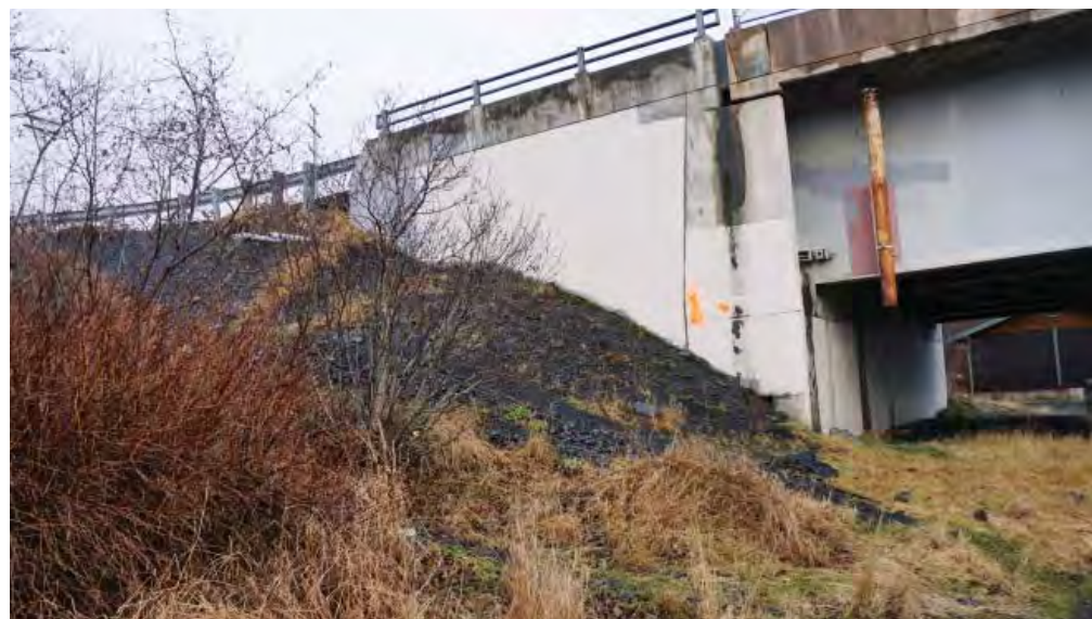
Image 28: West side of the bridge abutment.
