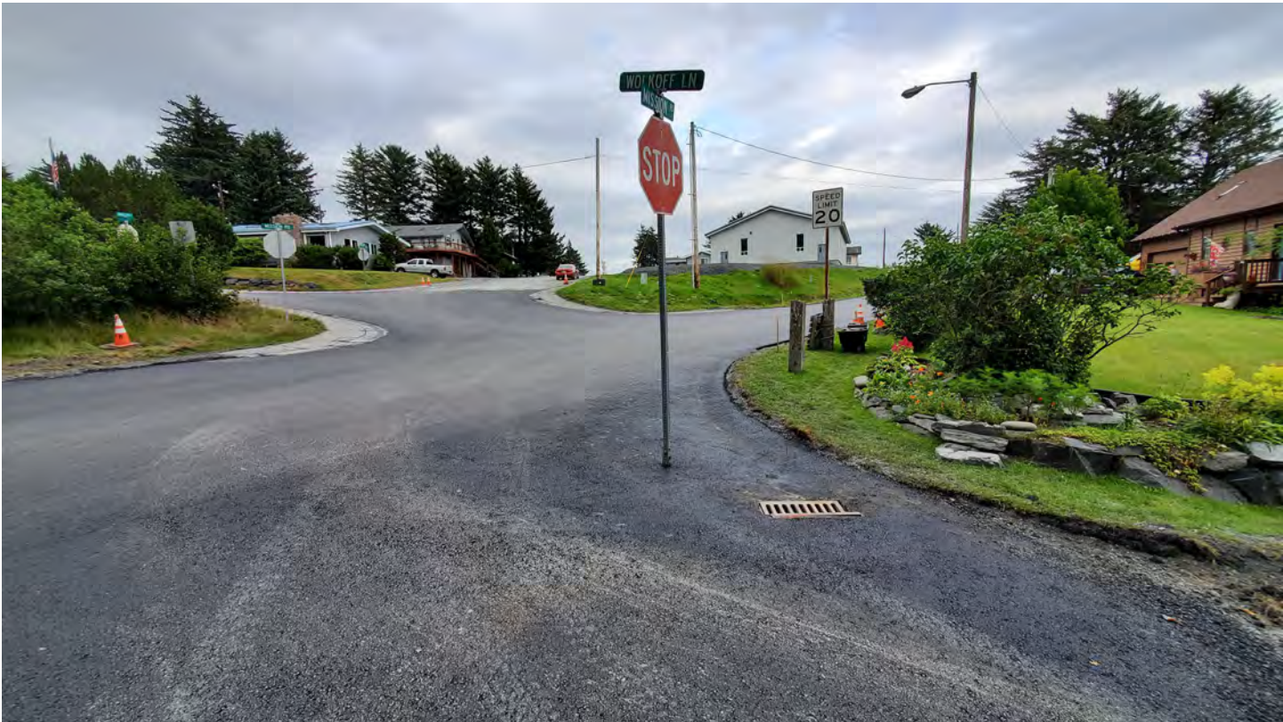
Mission Rd - New pavement, drainage improvements and sign
