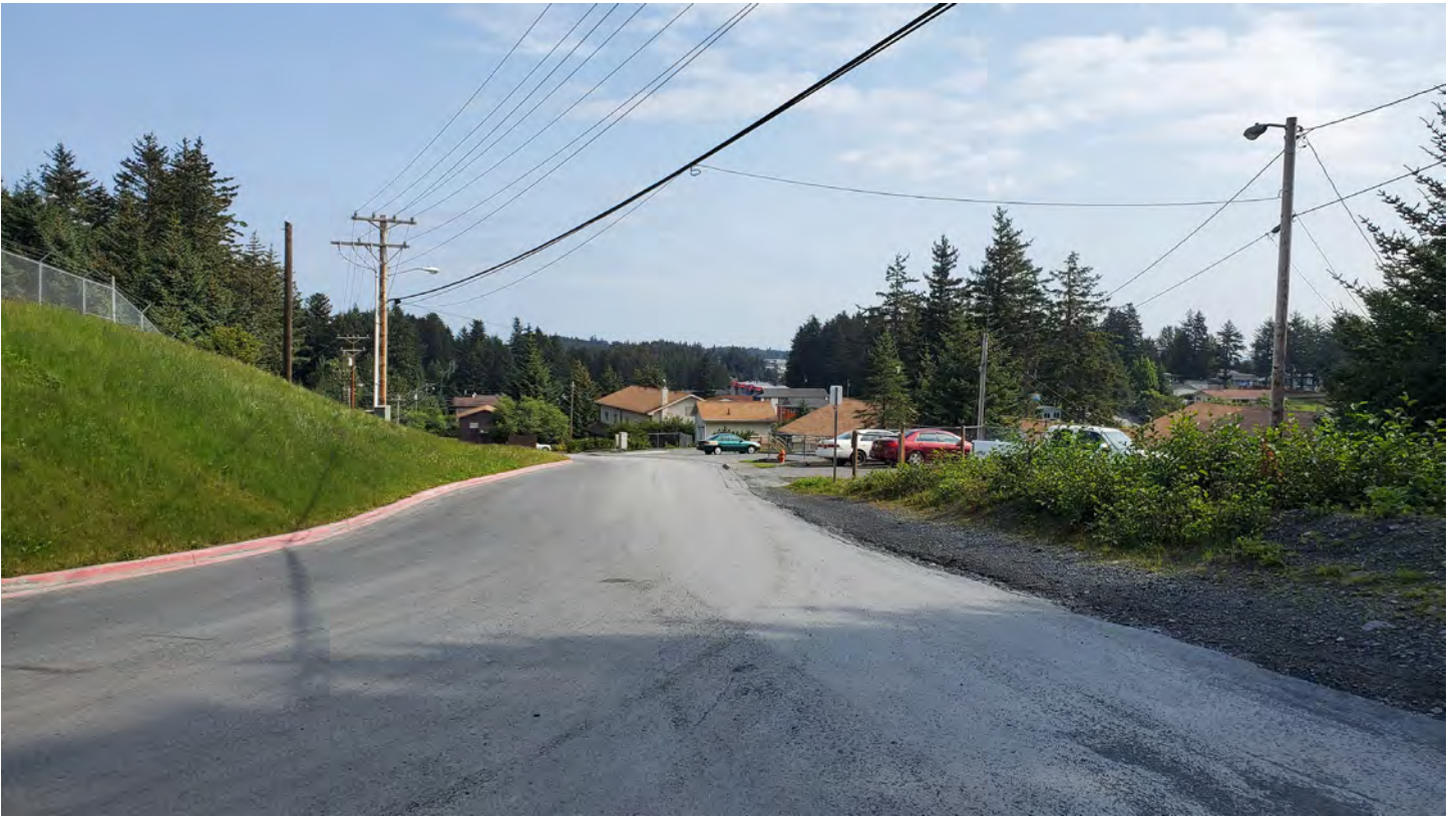
Pillar Mountain Rd (paved section)
