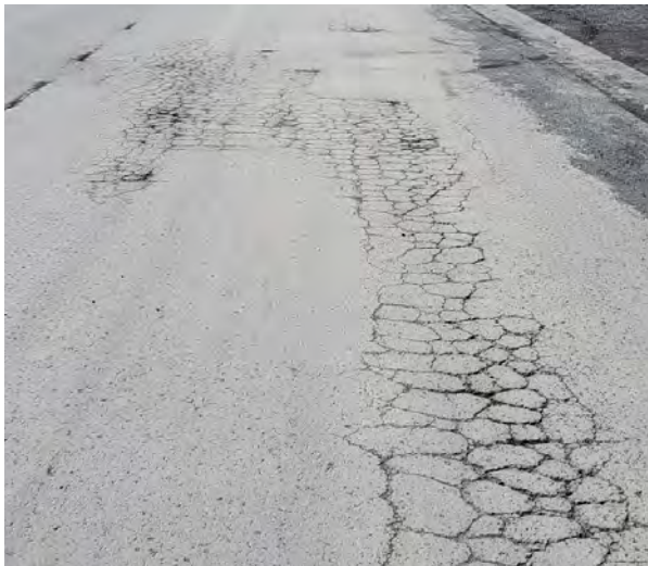
Left: Alligator cracking along East Marine Way. Right: Gravel portion of East Marine Way.
