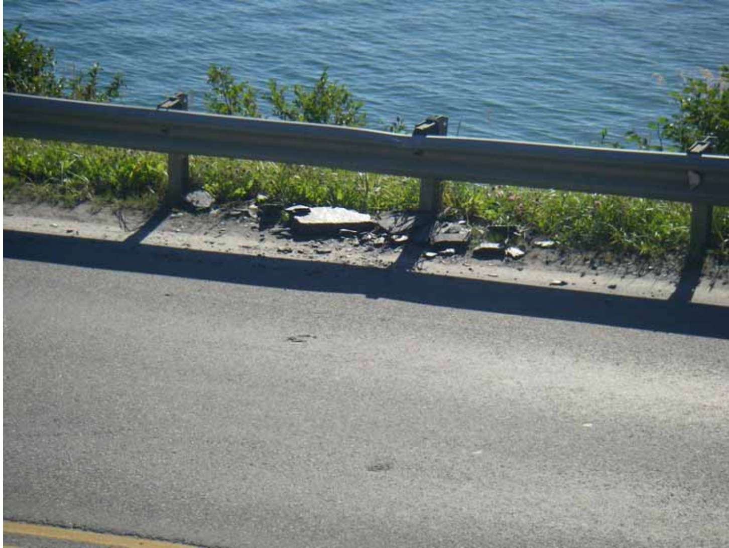
Rockfall across Road and Impact Craters on Pavement (September 21, 2013)
