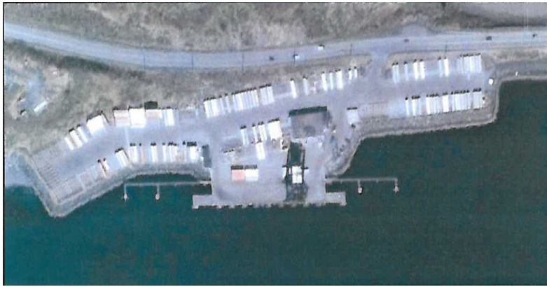
Aerial View of Pier III
