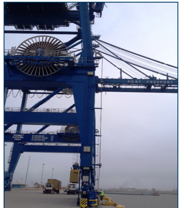
Sister Crane to new Kodiak Crane
