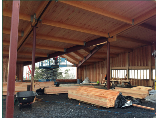
Contractor continues to install roof decking for the library.
