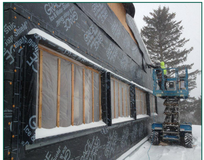
Contractor installing watershield barrier on building exterior.
