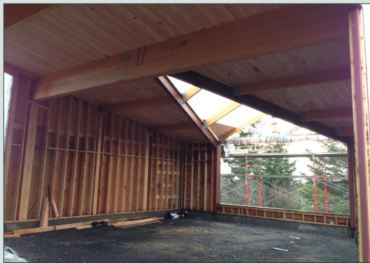
Framing the dormer above the multi-purpose room.
