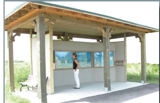
Covered information center/kiosk.
