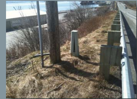
Guardrail and utility poles on Rezanof Drive.
