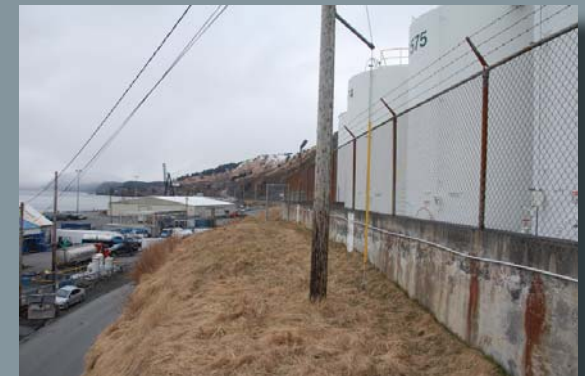
Fuel tanks on top of the bluff above Shelikof Street.
