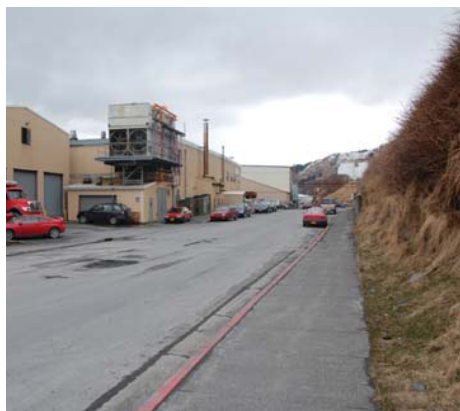
No parking zone delineated by red curb.
