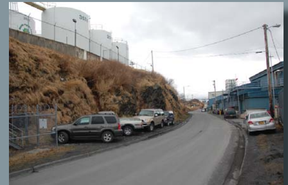
Rock bluff along north side of Shelikof Street.
