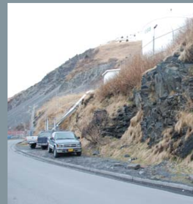
Parking over the existing curb.
