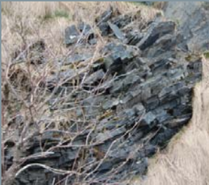
Close up view of rock face.
