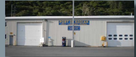
Port of Kodiak: Pier 2.
