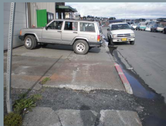
Parking over the existing sidewalk.
