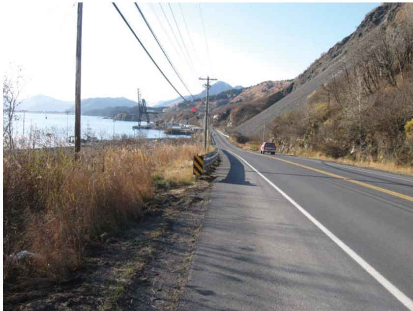
Rezanof Drive: south side between Pier 2 and Jack Hinkel Way.
