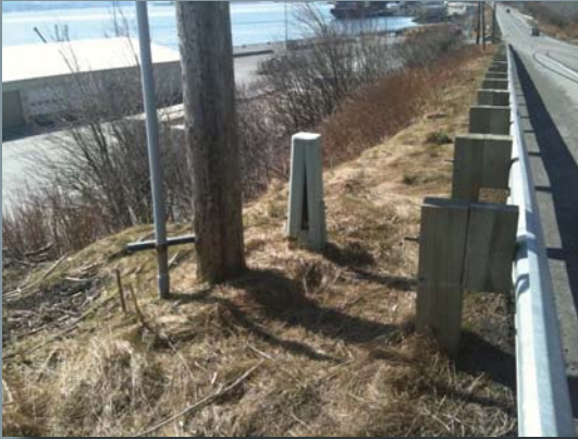
Utility pole near guardrail on Rezanof Drive.
