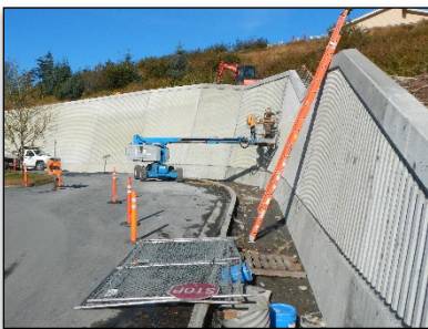
Completed Wall Sections
