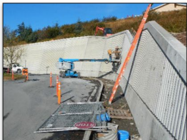
Completed Wall Sections
