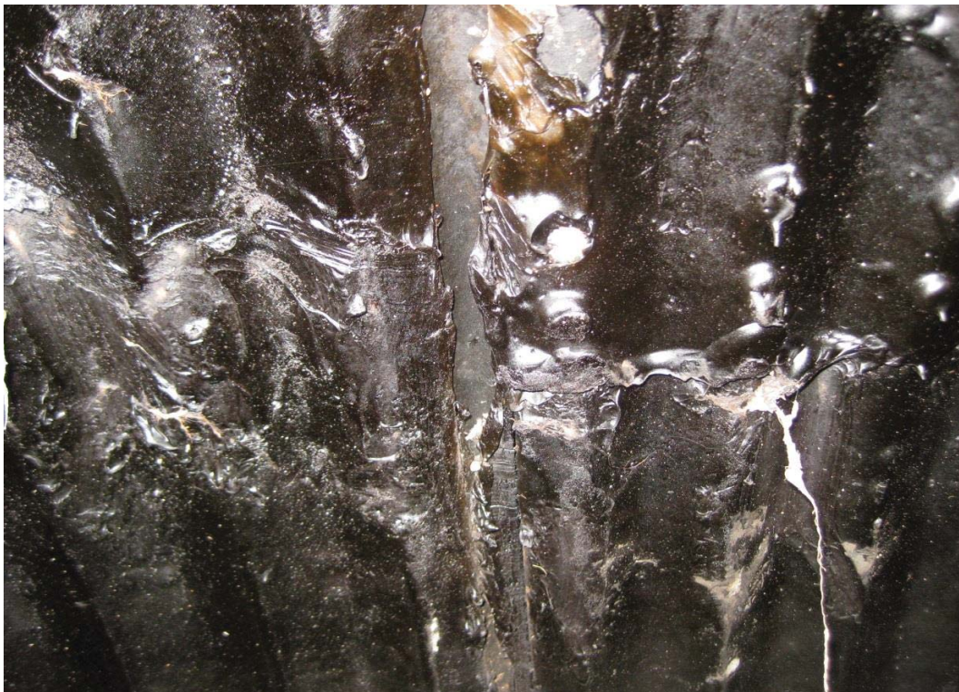
Drain A - 9' Seam at 10 o'clock with gap to 1-1/4".
