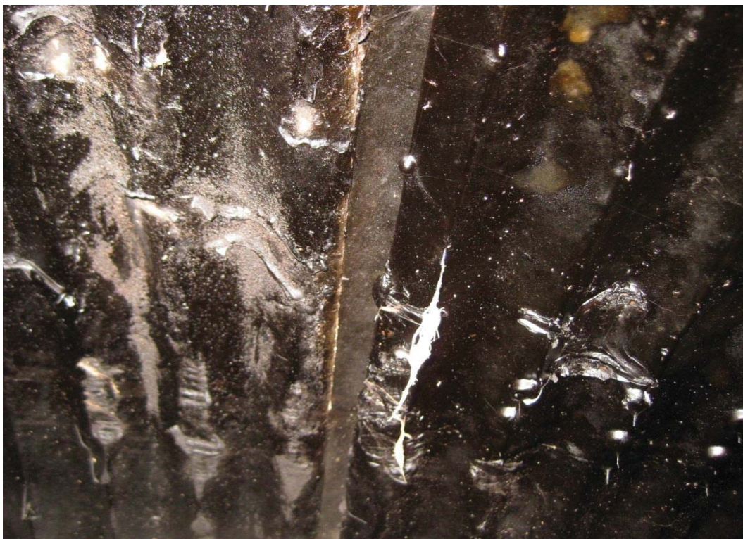
Drain A - 92' Seam at 9 o'clock with gap to 1-1/4". No corrosion or offset.
