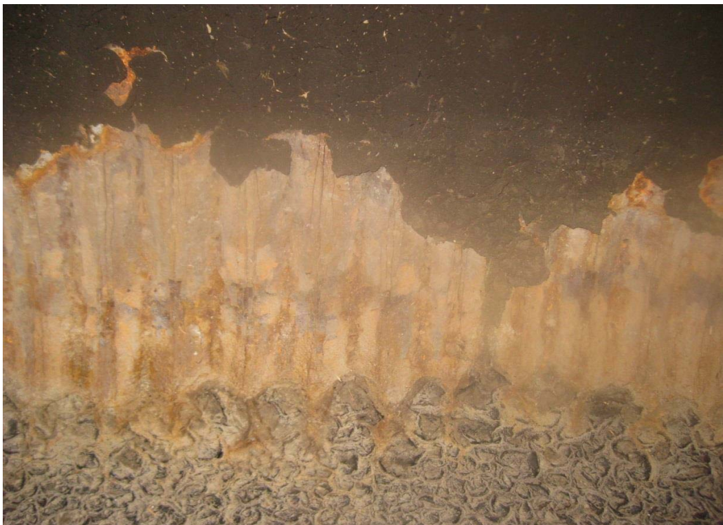
Drain A - 560' 2' coating failure with heavy corrosion to end of drain at 9 o'clock and 3 o'clock.
