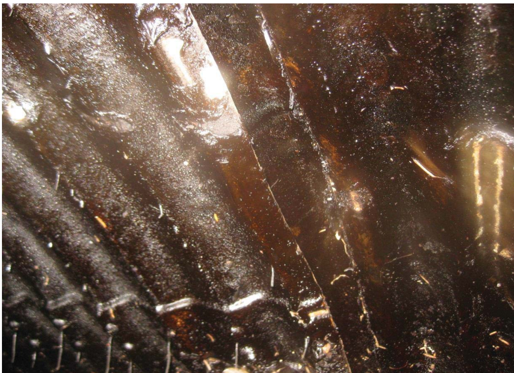
Drain A - 541' Seam at 9 o'clock looking upstream with gap to 1-1/2" and an offset of 2".
