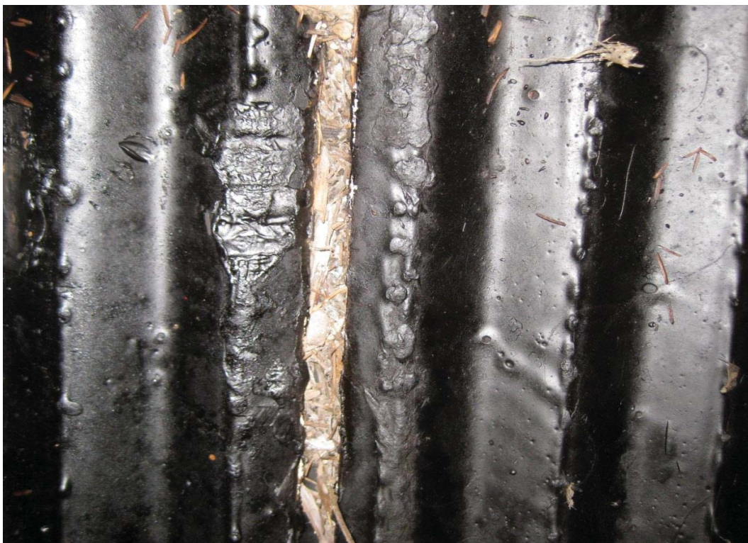
Drain A - 225' Seam at 12 o'clock with gap to 1" and offset up to 1/2".
