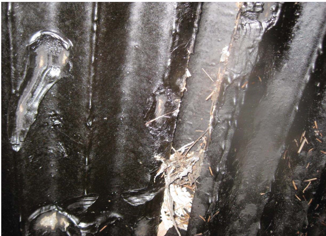
Drain A - 247' Seam at 3 o'clock with gap to 1-1/2". No offset or corrosion.
