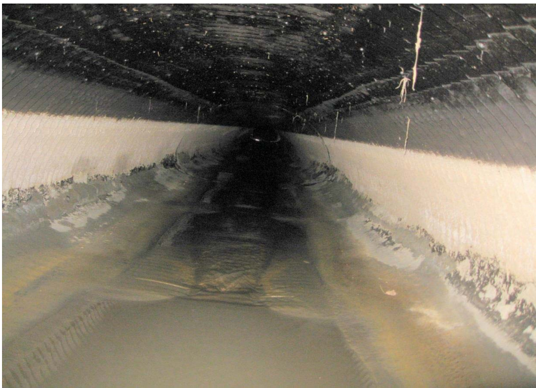
Drain B - 400' View downstream. Coating is intact.
