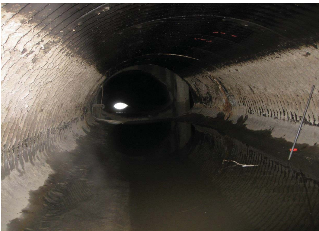
Drain B - 495' View downstream. Drain is half full of tidewater. Coating is thin.
