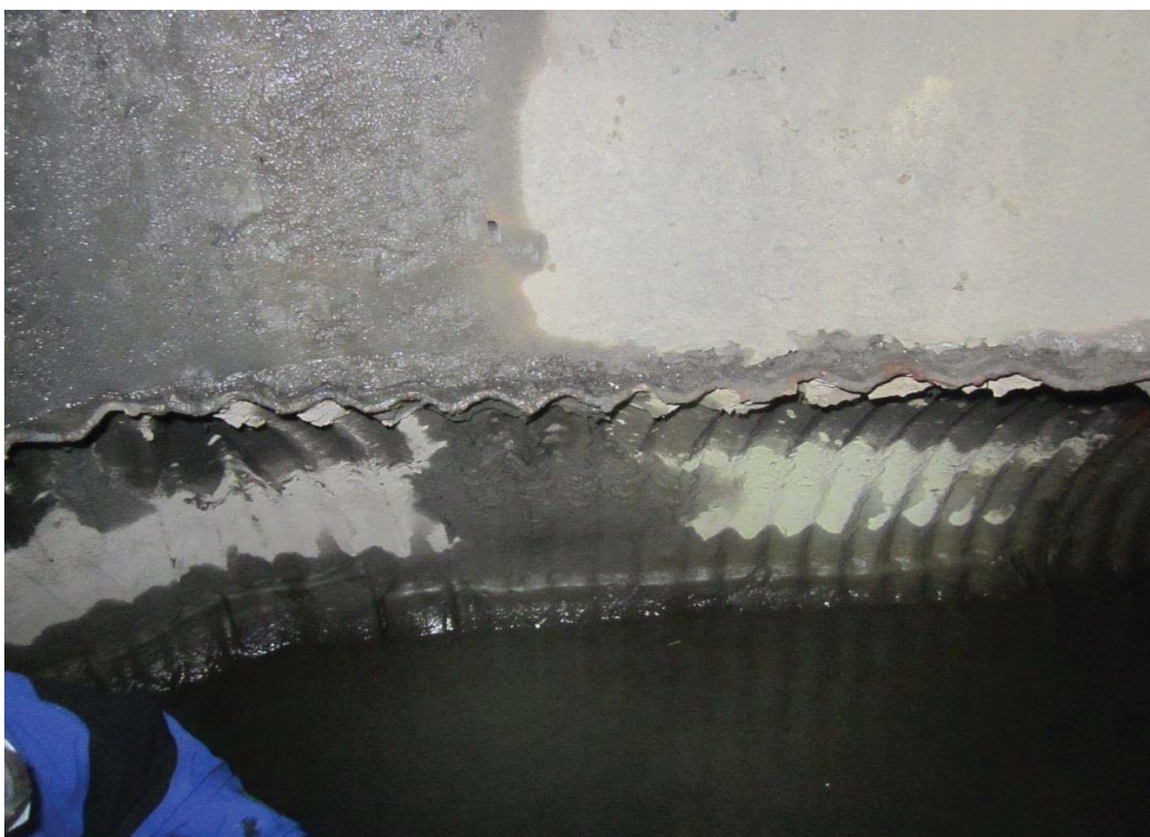
Drain B - 140' Seam beneath manhole at 9 o'clock. No significant deficiency.
