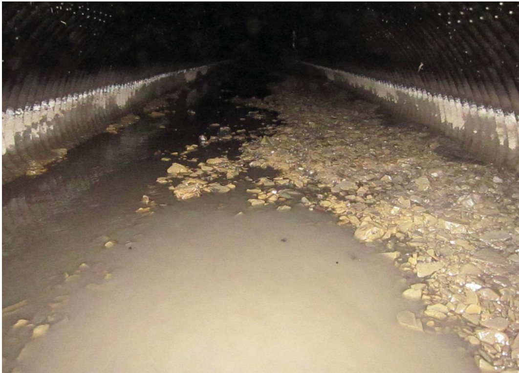
Drain B - 50' View downstream from culvert. Up to 1' of sand and rock deposits.
