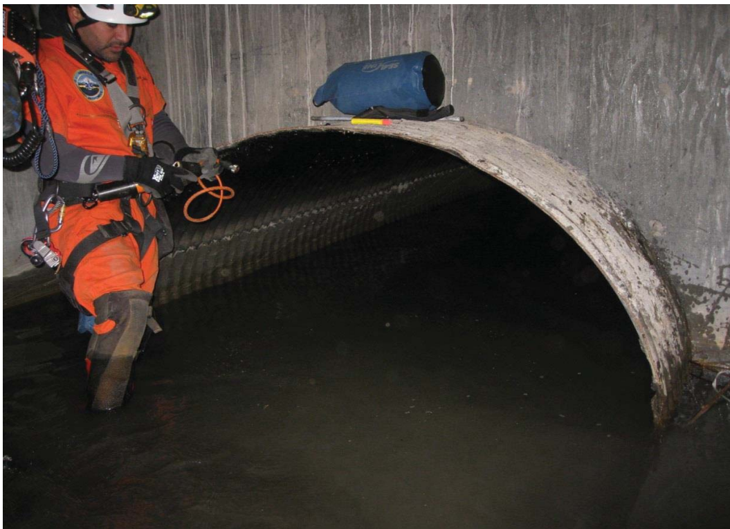
Drain B - 0' Ultrasonic testing location at entrance to Drain B. Some damage to coating on torch cut edge. Sandy soil in bottom.
