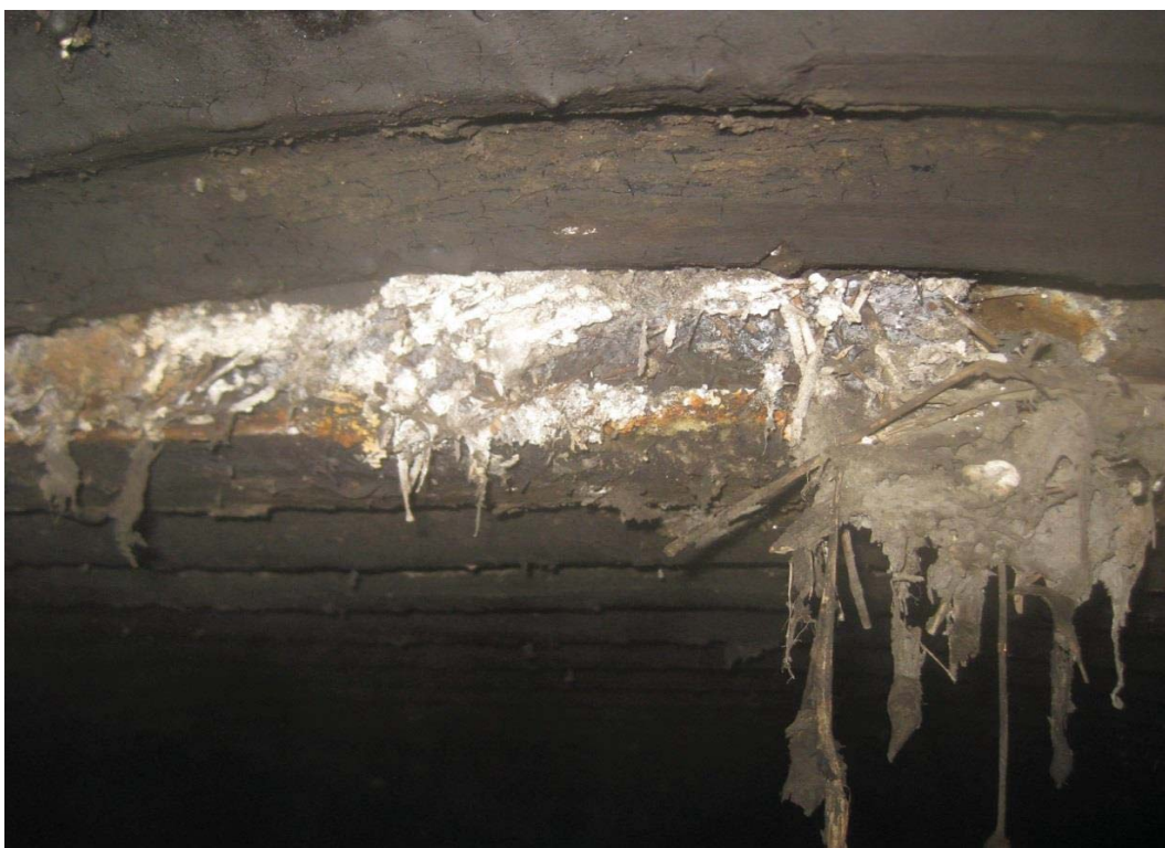
Drain A - 487' Seam at 12 o'clock with gap to 1" and an offset of 1-1/2".
