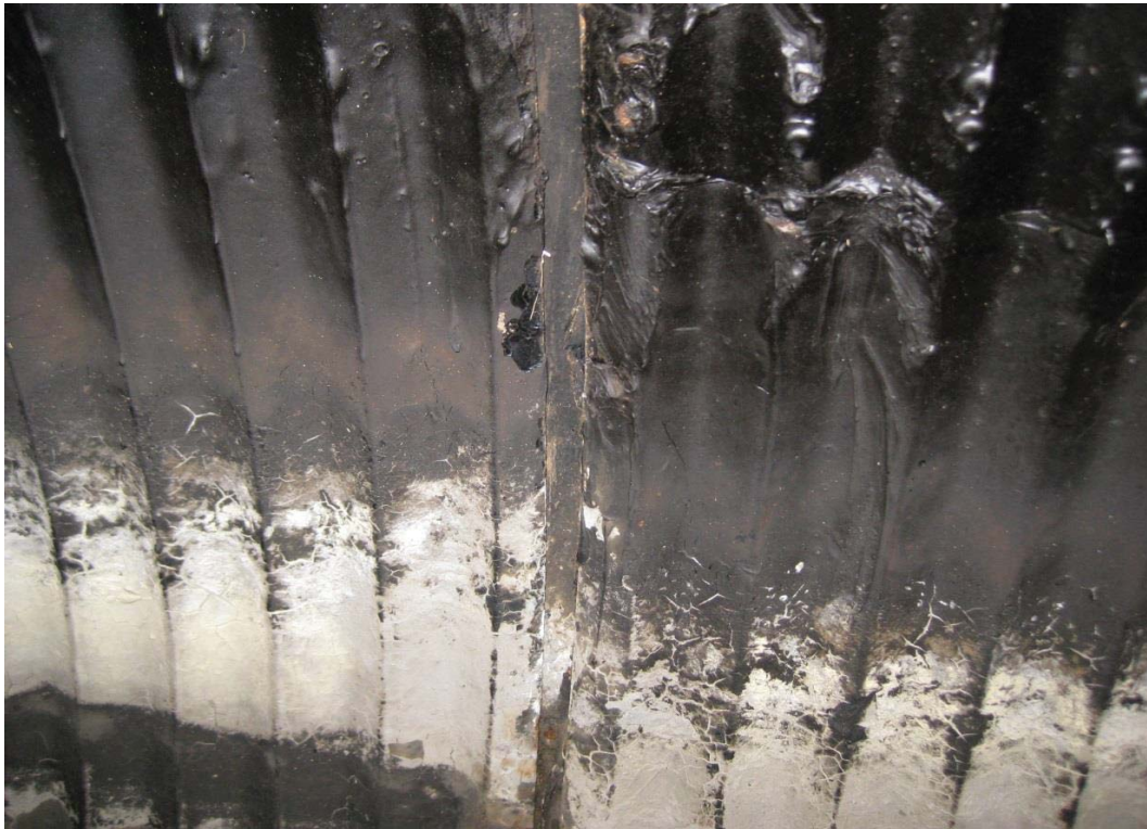
Drain A - 9' Seam at 9 o'clock with gap to 1".
