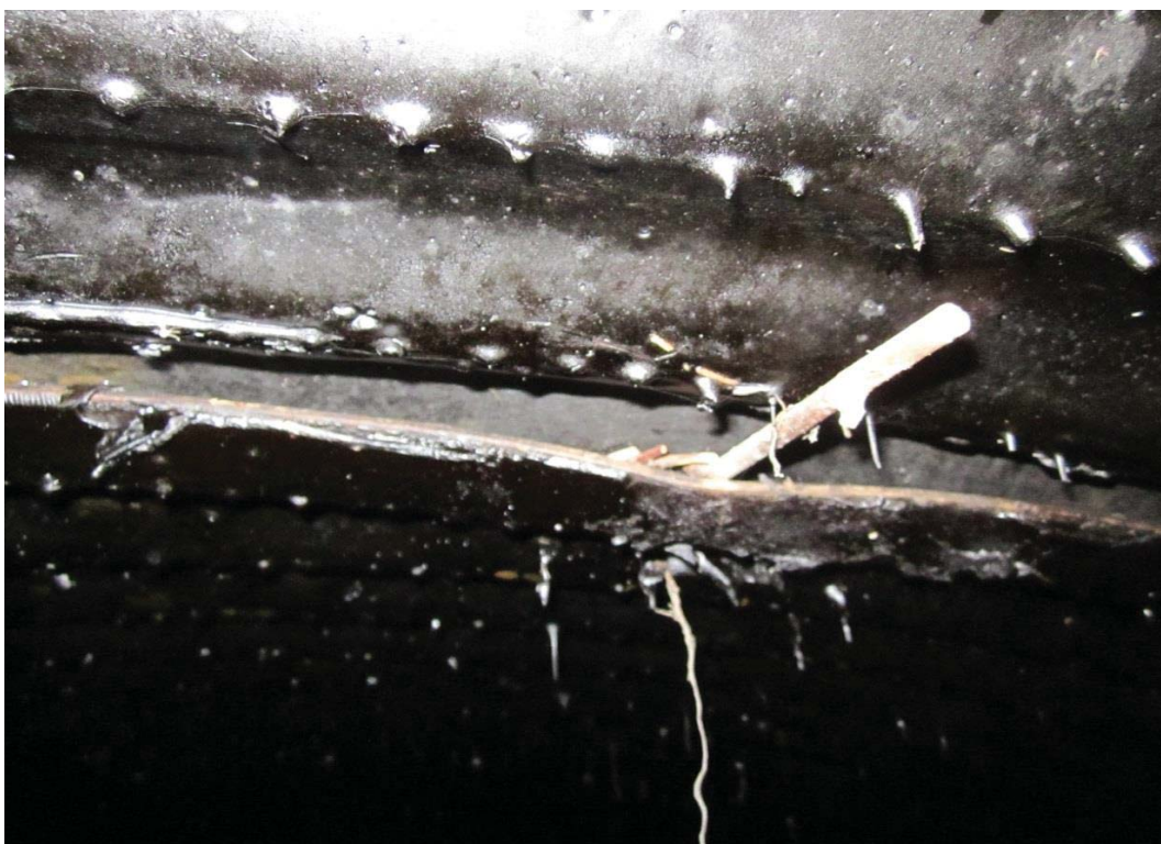
Drain B - 70' Seam with gap to 1" and opening of 7".
