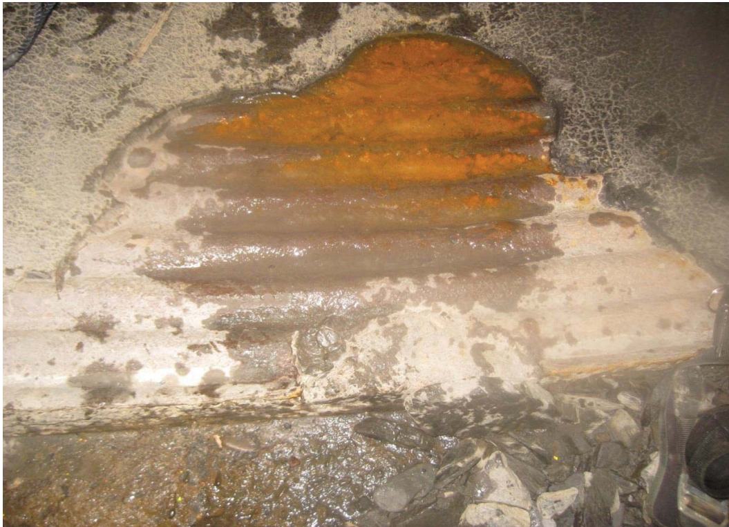
Drain A - 521' 2' x 2' area of failed coating at 6 o'clock with moderate surface rust.
