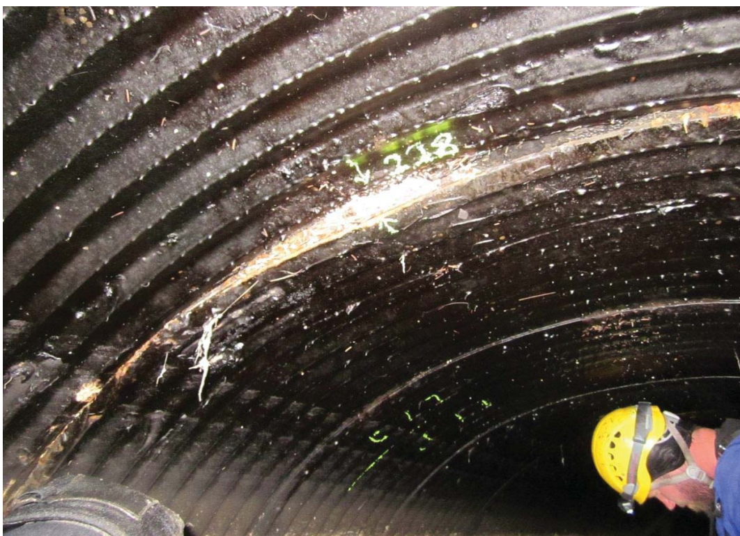
Drain B - 228' Seam at 12 o'clock open to 1-1/2" with offset of 1-1/4". Minor coating damage on edge with surface rust.
