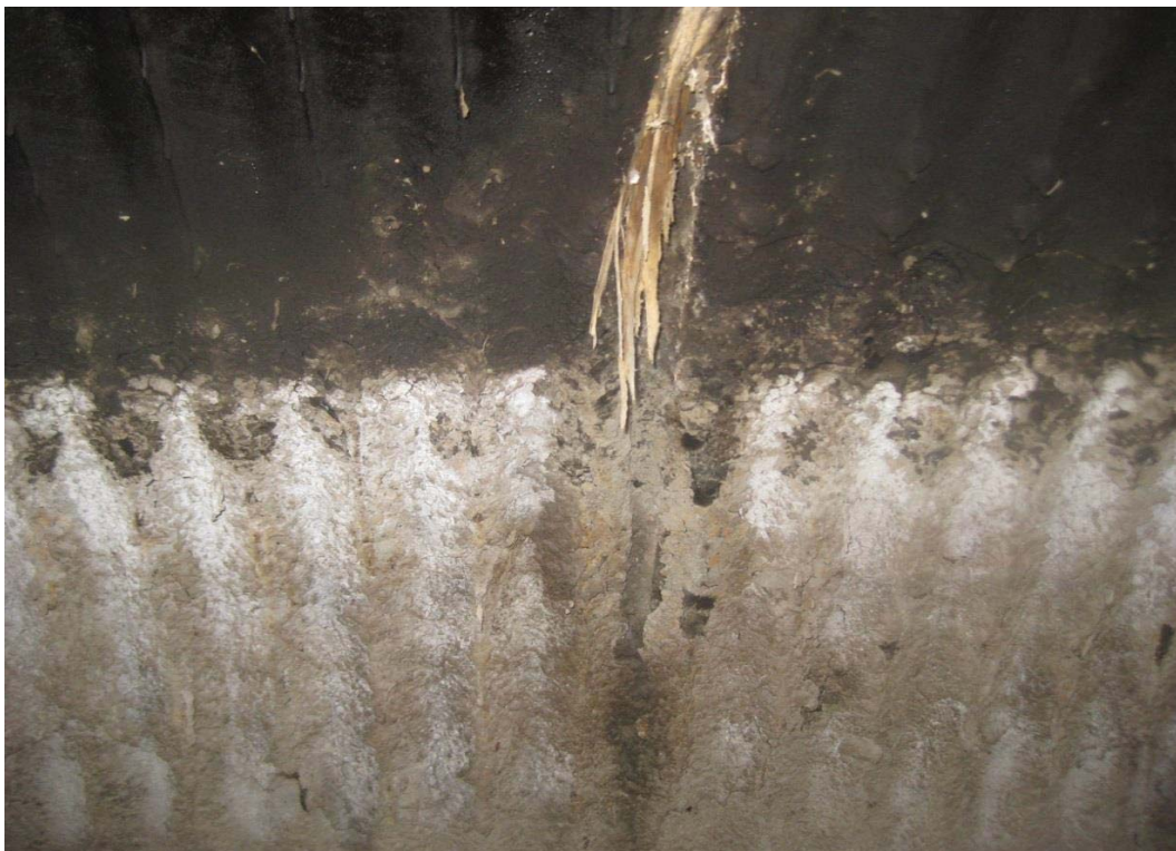
Drain A - 466' Seam at 9 o'clock with gap to 1-1/2" and an offset of 1". Moderate corrosion.
