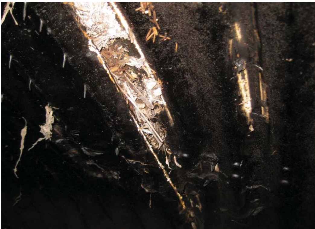
Drain A - 113' Seam at 9 o'clock with gap to 1/2" and offset of 1-1/2". Minor corrosion on edge.
