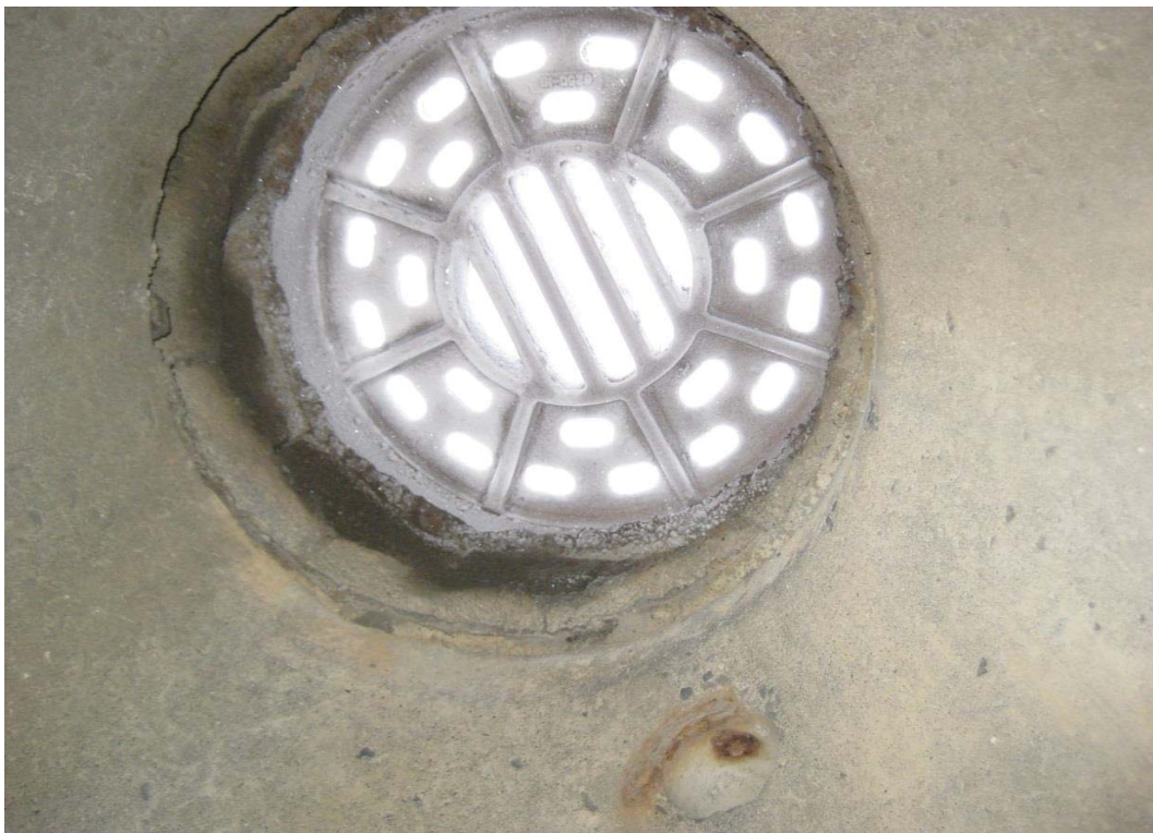
View of 12 o'clock position. 46" torch cut hole with moderate surface rust on the edges. View is looking up at cast iron manhole cover. This manhole is at the bend in the drain. No significant deficiency.
