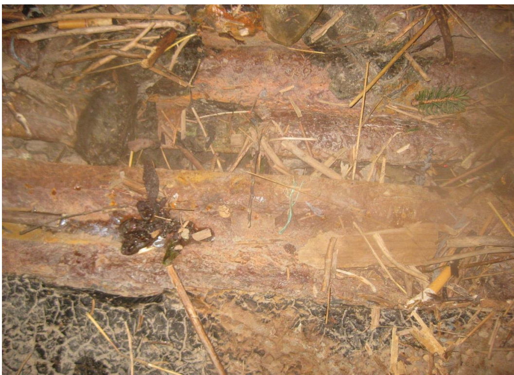
Drain B - 557' Seam at 6 o'clock with gap to 1" and offset up to 2". Heavy corrosion.
