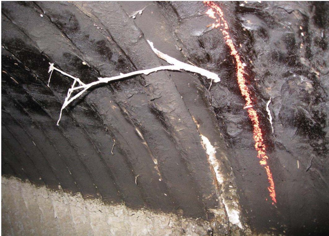
Drain B - 424' Seam at 1:30 with vertical gap to 1/2" and horizontal gap to 1".
