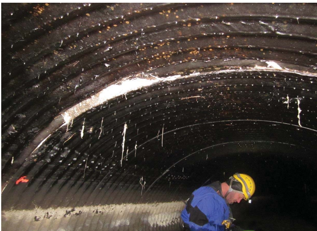
Drain B - 268' Seam with gap open to 2" with offset of 1" at crown.
