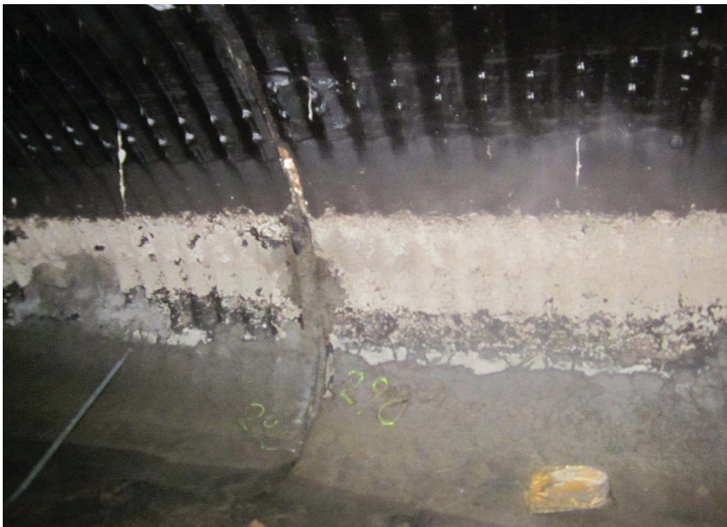
Drain B - 290' Seam with gap open to 1-1/2" with water flowing out at the 7 o'clock position. Flow rate is approximately 2 gallons/minute.
