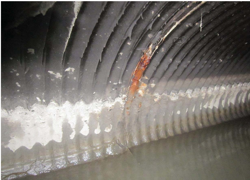
Drain B - 142' Seam open to 3/4" with minor surface rust and coating damage.
