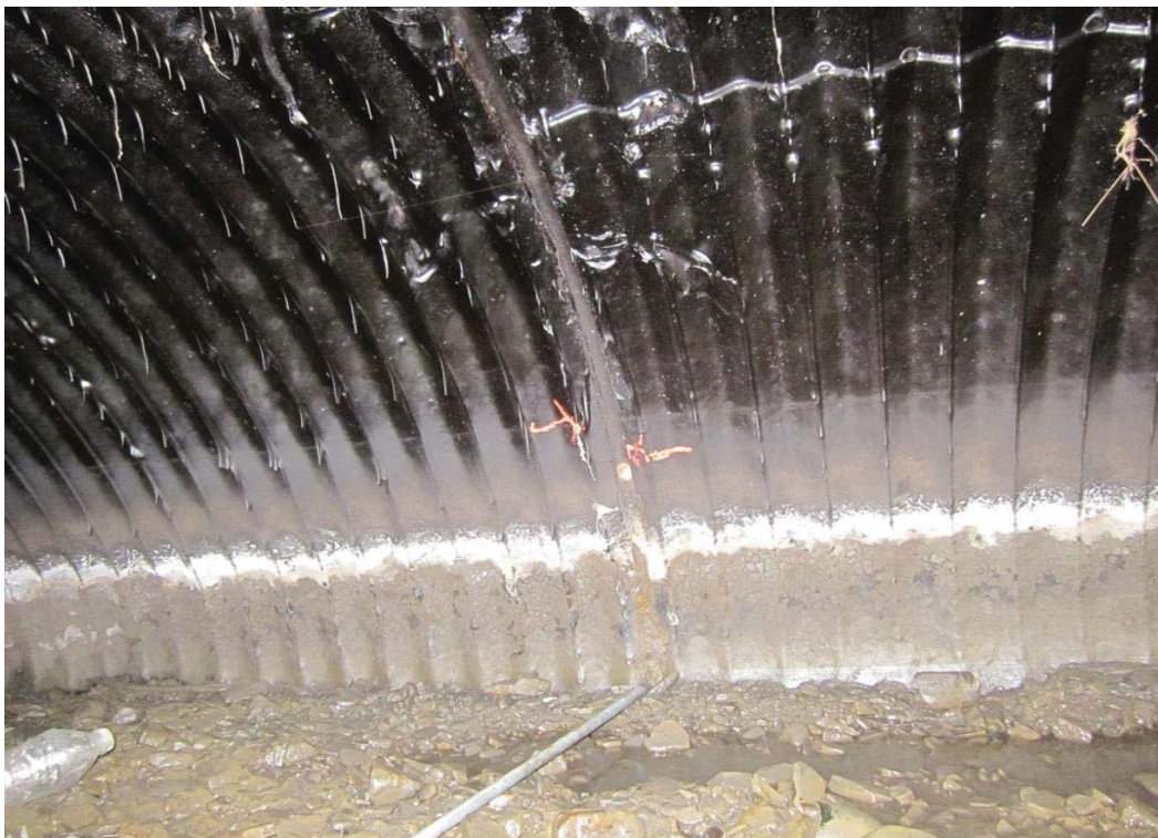
Drain B - 90' Seam open to 1-1/2".
