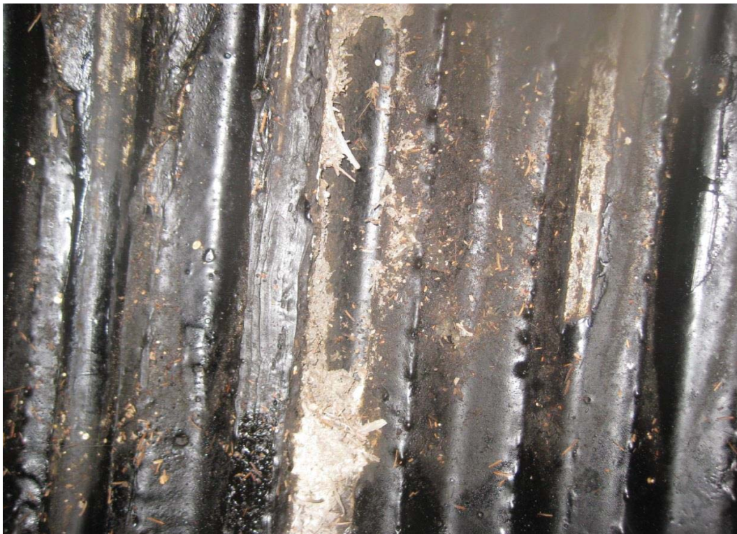
Drain A - 380' Seam at 12 o'clock with gap to 2" and an offset up to 1/2".
