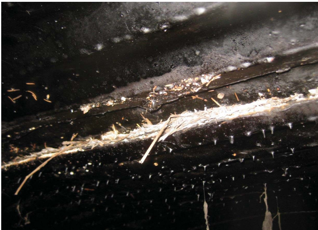
Drain A - 288' Seam at 12 o'clock with gap to 1" and an offset of 2". There is a 2' square area that is caved or pressed in 2".
