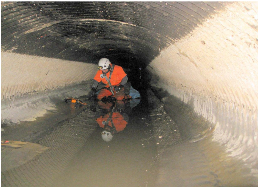
Drain B - 495' looking back at 484'. View upstream. Ultrasonic testing and coating removal.
