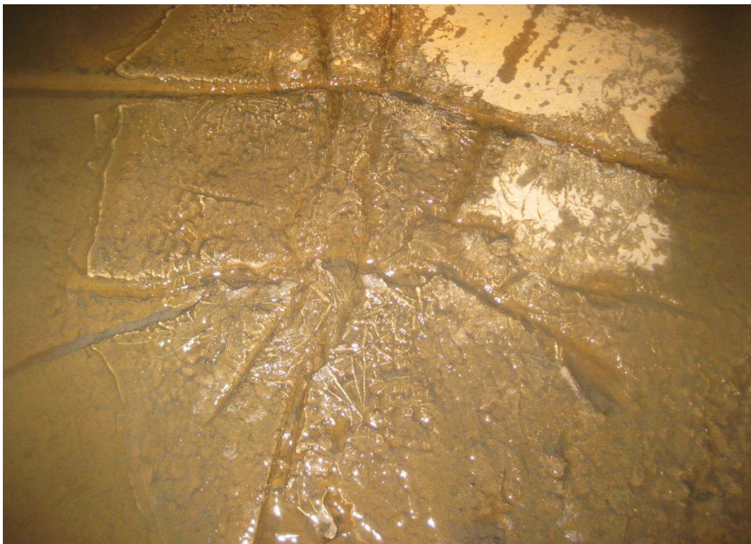
Drain A - 497' View of 3' x 2' x 2" caved in area at 6 o'clock for 2".
