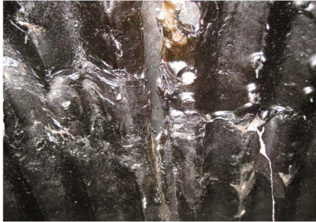
Photo 1 - Drain A - Separated joint showing no corrosion or signs of leakage
