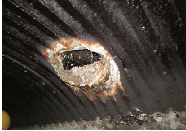
Photo 9 - Drain B - Flame cut inlet opening
